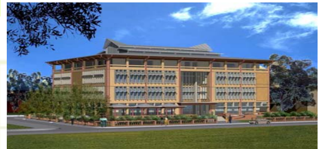
Hue LRC, now under construction
